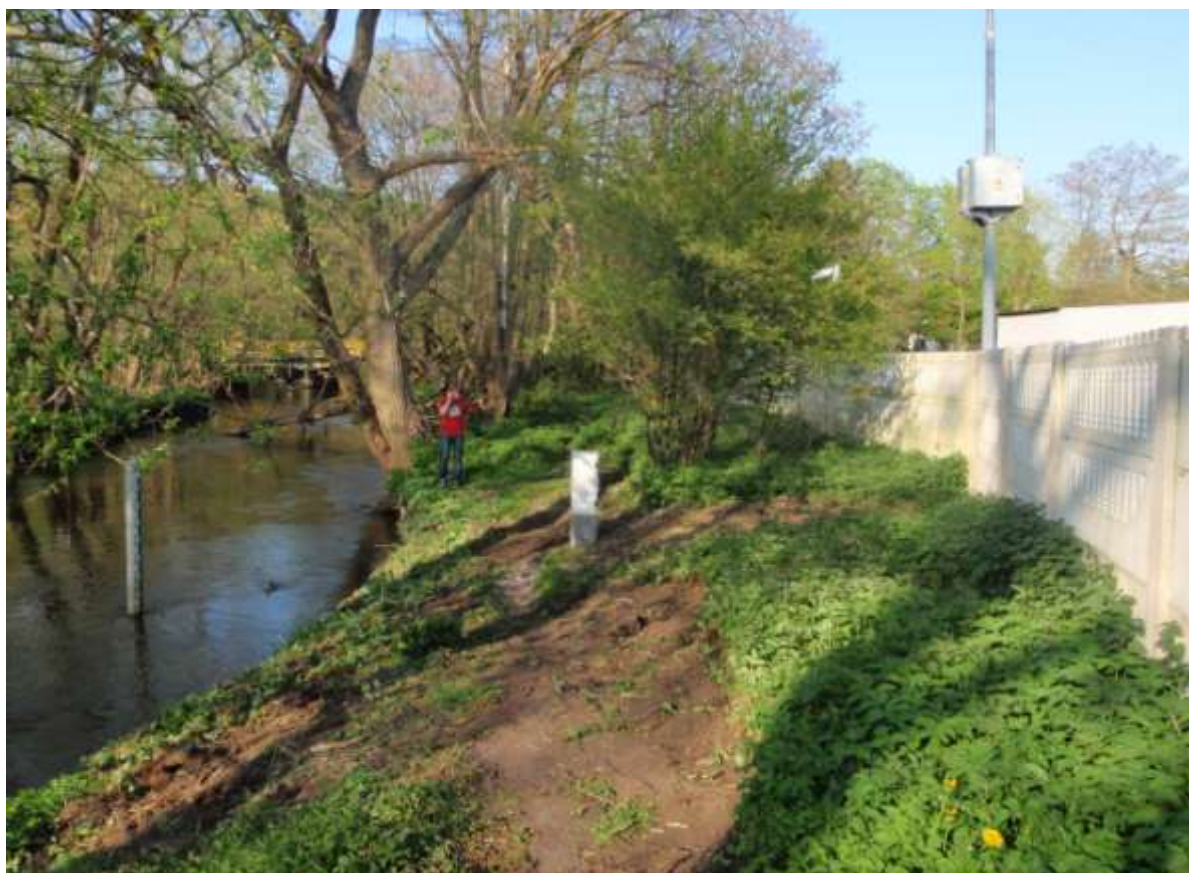
Photo. Installation of the spectrometer type S: Can Nitro: lyser in Reda river
